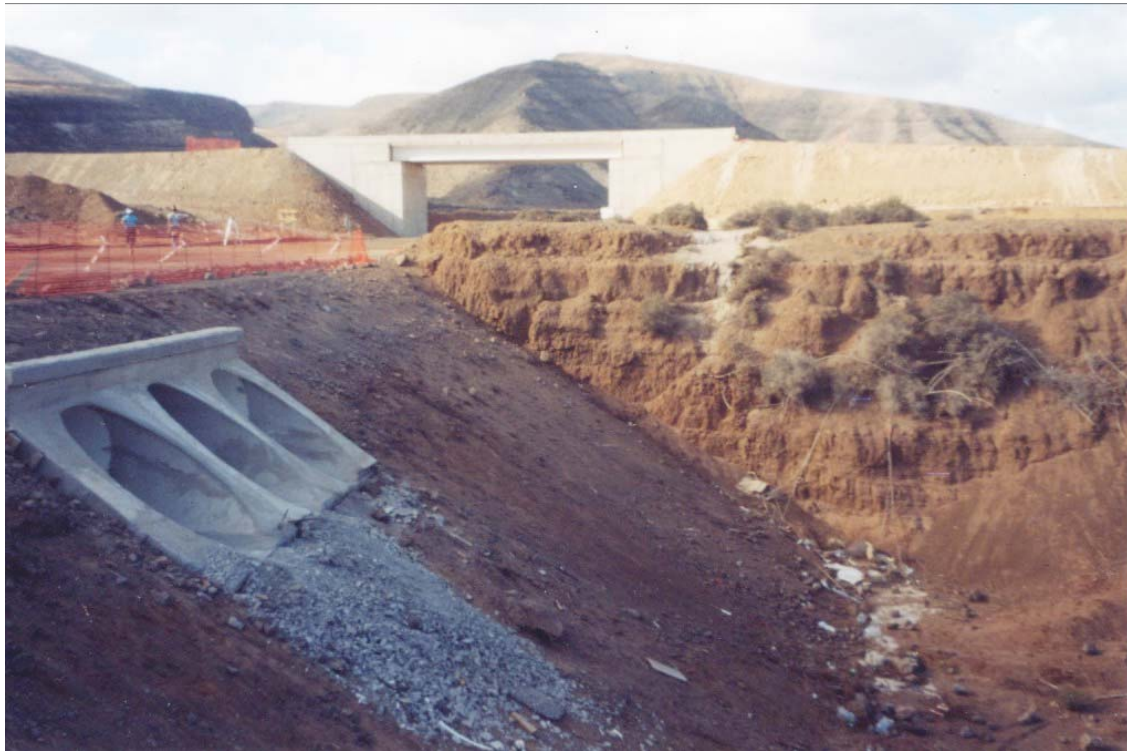
Figure 2: View of the “Guatiza II” exposure. The profile in which the ovicaprid bone was found is now masked by the road dam. By February 2003, the site had already been destroyed (photo: H. v. Suchodoletz).
