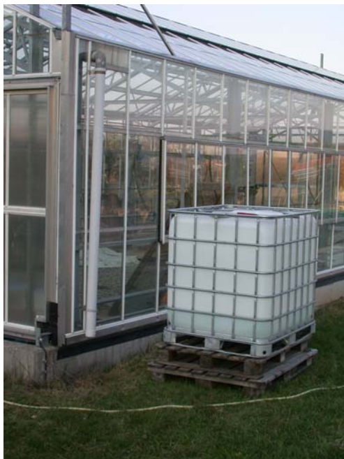
Figure 15 Container for storing precipitation water, collected from the roof of a greenhouse
