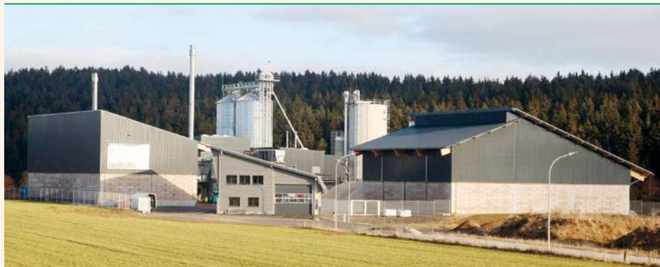
■ Fig. 2: Wunsiedel Energy Park will combine renewable energy sources, an electrolysis plant (power-to-gas plant still under construction) for the production of "green" hydrogen, combined heat and power plants, and industrial production (wood-pellet production) (Photo: SWW Wunsiedel).
