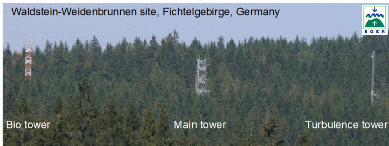
Figure 4: Towers at the Waldstein-Weidenbrunnen site: the 36 m high ‘bio tower’, the 32 m high ‘main tower’ and the 35 m high ‘turbulence tower’ (from north-west to south-east, photo by J. Lüers).
