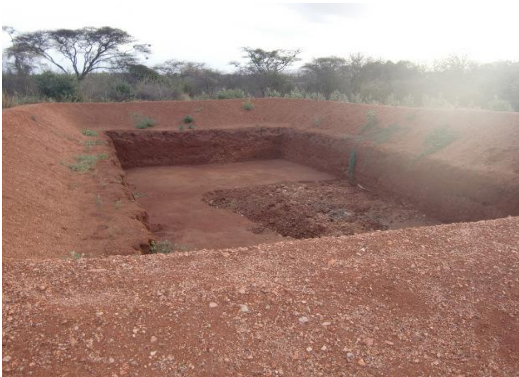
Photo 25: A privately owned earth dam under construction
