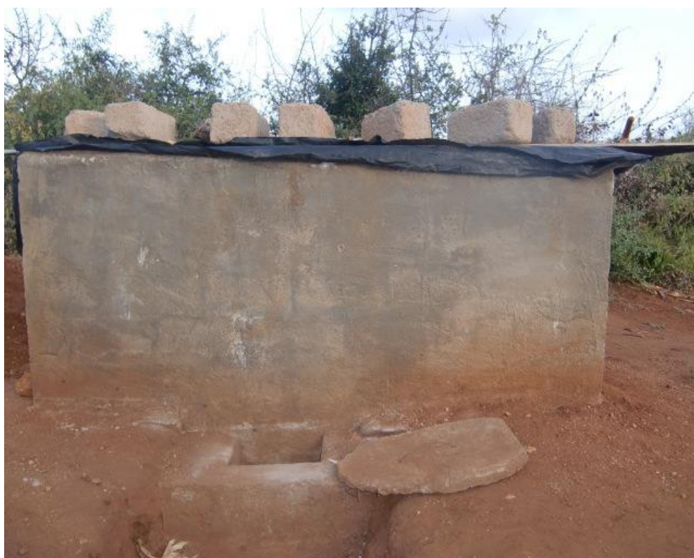
Photo 26: A run-off water collection tank
