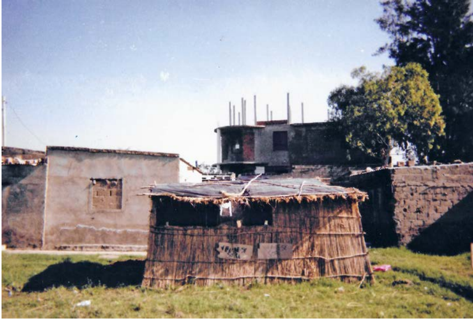
Photo 7 Peri-urban construction materials and house types
