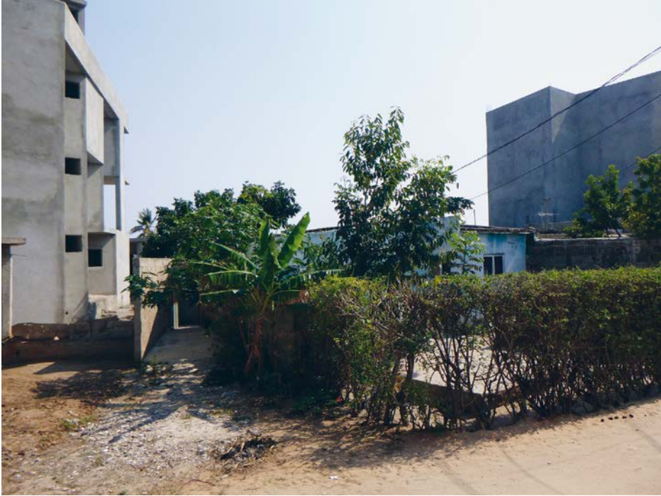
Photo 16 Senhor Bernardo's home surrounded by buildings
