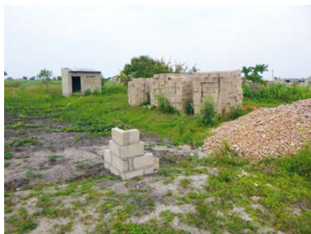
a) Piles with cement blocks
