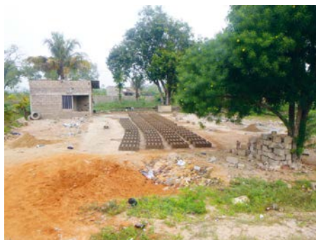
b) On-site construction
