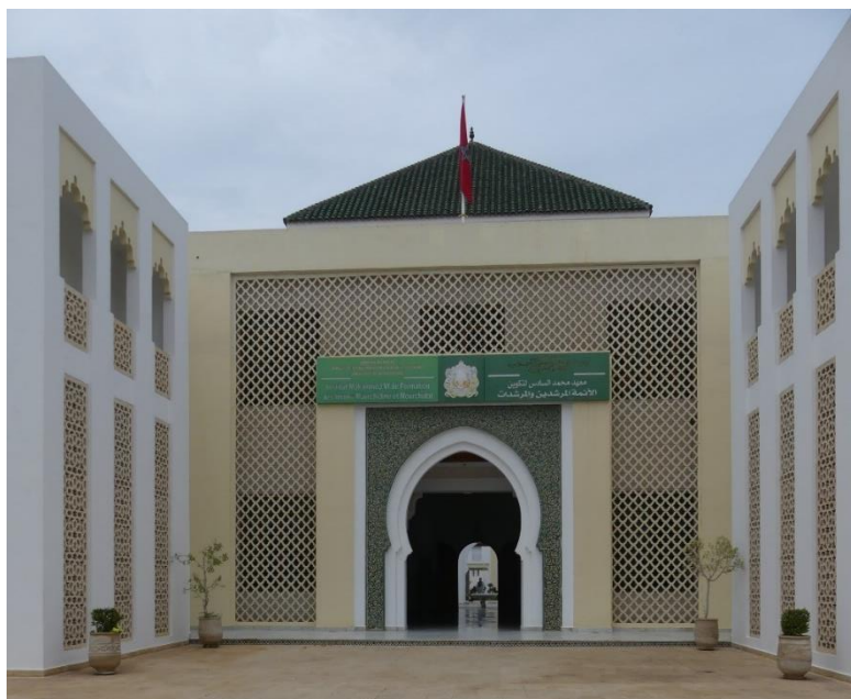
Figure 64: Main entrance to Mohammed VI Institute for the Training of Imams, Murshidin and Murshidat
