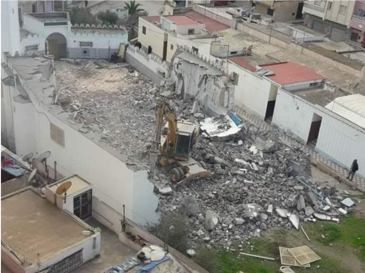
Figure 12: Demolition of the Mohammed V mosque in al Hoceima 134
